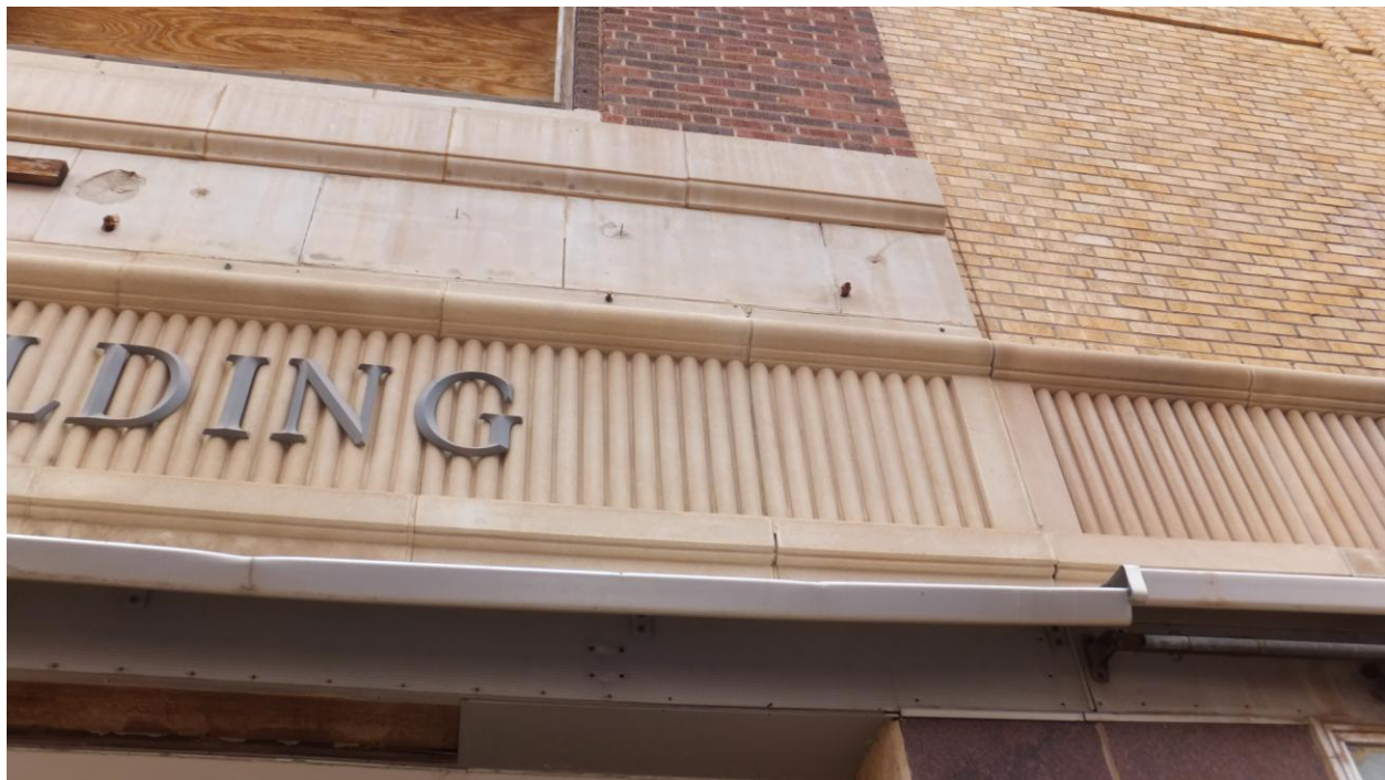
Photograph showing the decorative stonework, contrasted with the later addition of a cast stone ribbon which was added to tie the 1949 addition architecturally to the original.
