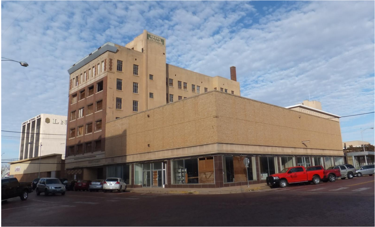
Existing Building Condition
