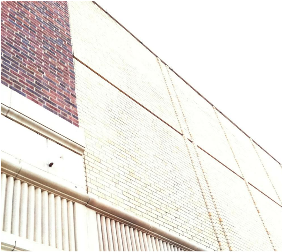
Photograph showing stacked header bond on the 1949 addition
