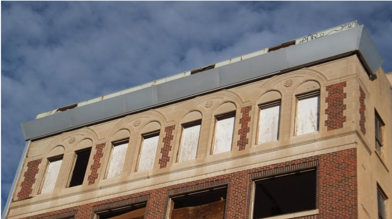
Photograph showing the Neo-Classical Revival features of the sixth story (decorative stonework, quoining, simple entablature, faux balustrade covered in the metal paneling)
